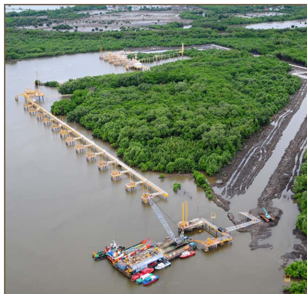
Operations close to mangroves (new trench ROW full of water at high tide).
