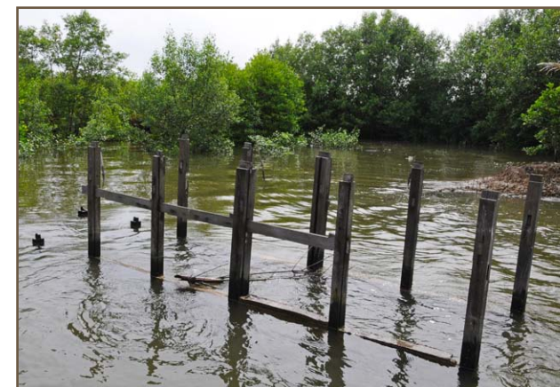
When the shrimp pond doors are not maintained, mud dykes are quickly destroyed. Water can then easily penetrate the pond and the tidal cycle is restored.
